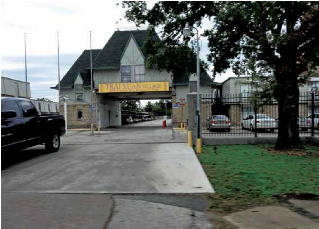
The Thai Xuan Village condominiums along Broadway have struggled to fund needed maintenance.
