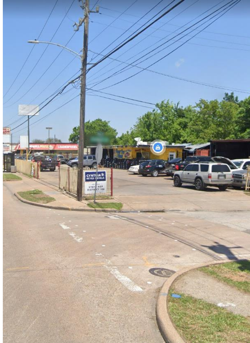
Lack of Ped Ramps
