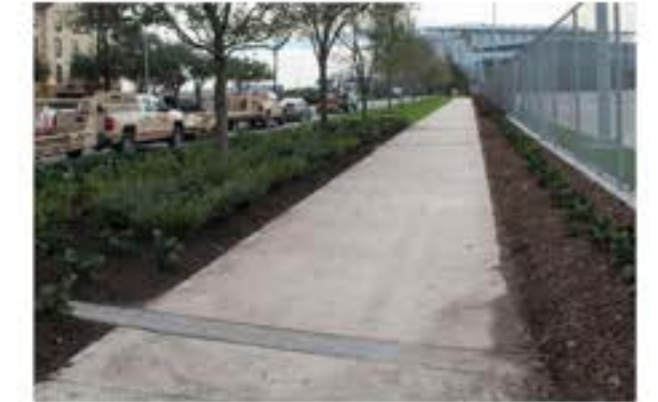
01_ 6' GRAY CONCRETE SIDEWALK
