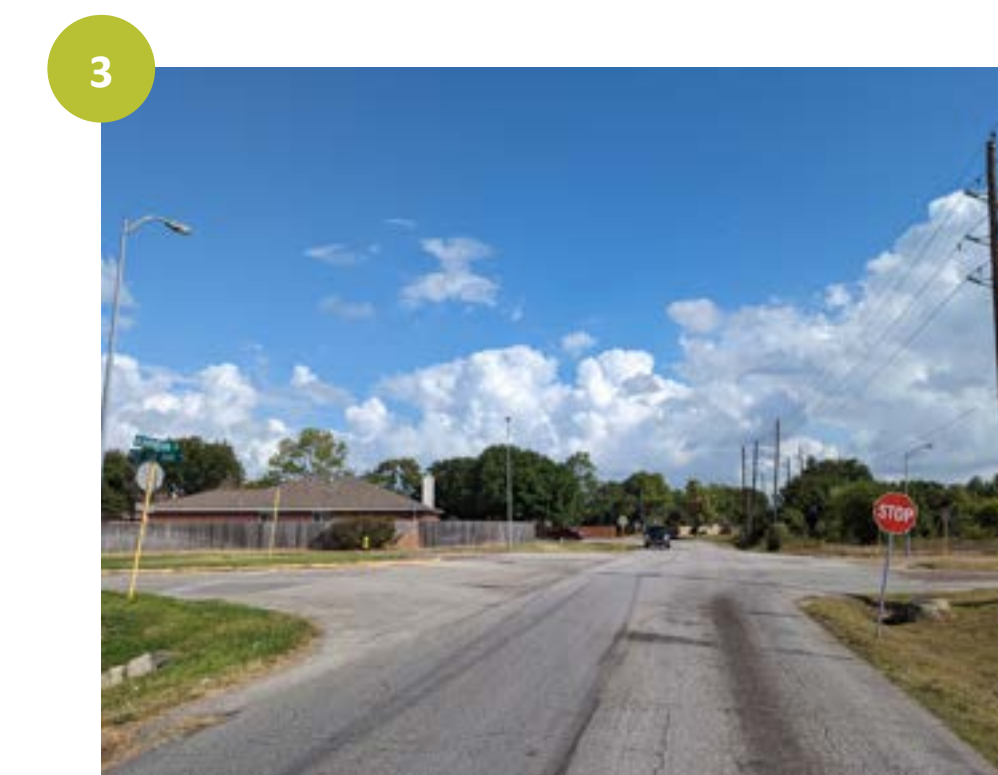
3 Intersection of West Gulf Bank Road & Alabonson Road
