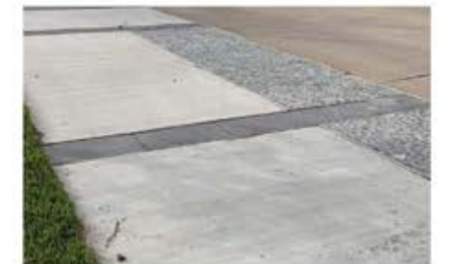
03_ SANDBLASTED DARK GRAY UPGRADED CONCRETE BAND
