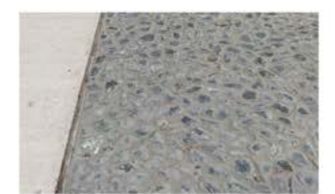
04_ MORTARED AGGREGATE IN RAISED ISLANDS
