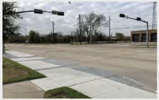
Completed sidewalk on W Little York
